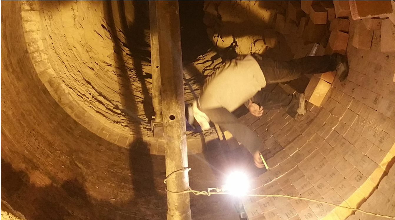
>> Annual maintenance of the Kiln - laying of the refractory bricks
